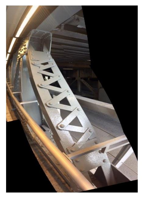
Project Details: City of Calgary - CP Rail Steel Bridge / Overpass encapsulation of lead-based paint and rust.
