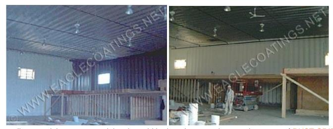
The walls around the room containing the acid bath tanks were given a primer coat of <u>RUST GRIP</u> ® first to protect against corrosive vapours.
