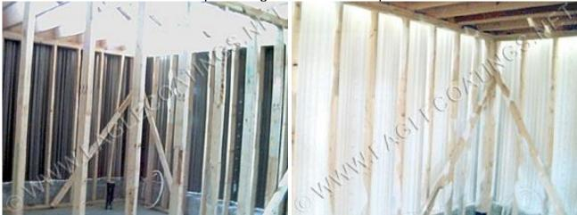
The ceiling above the acid bath tanks was also coated with <a href="RUST GRIP">RUST GRIP</a> ® only to protect against the corrosive vapour's.
