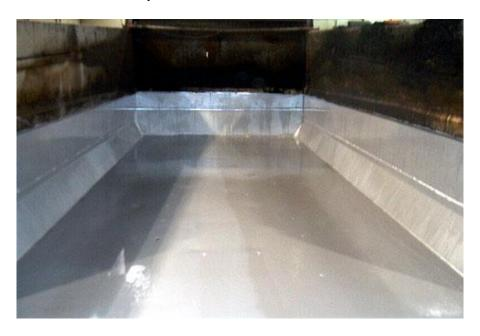
Because the <u>RUST GRIP</u> ® coating was done during the regular maintenance shutdown it was allowed in excess of two weeks to ensure maximum cure before going into service.
