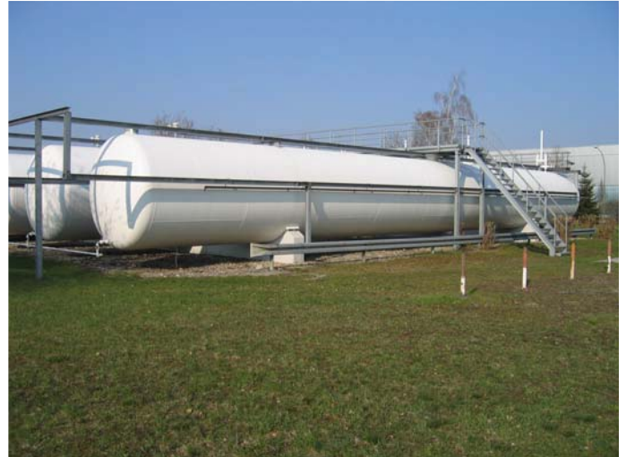
Germany – Liquid Gas Tanks After Coating Rust Grip® and Super Therm®
