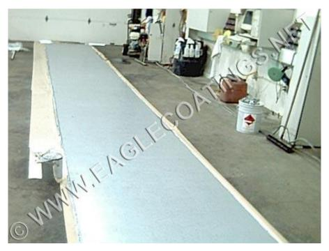
A less aggressive coating system than that used on offshore oil rigs was applied. A resin aggregate (less abrasive) was broadcast and back rolled into the primer coat of RUST GRIP (NS) ®.
