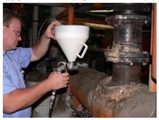
Surface Temperature after application to meet OSHA requirement 139°F \ 59°C
